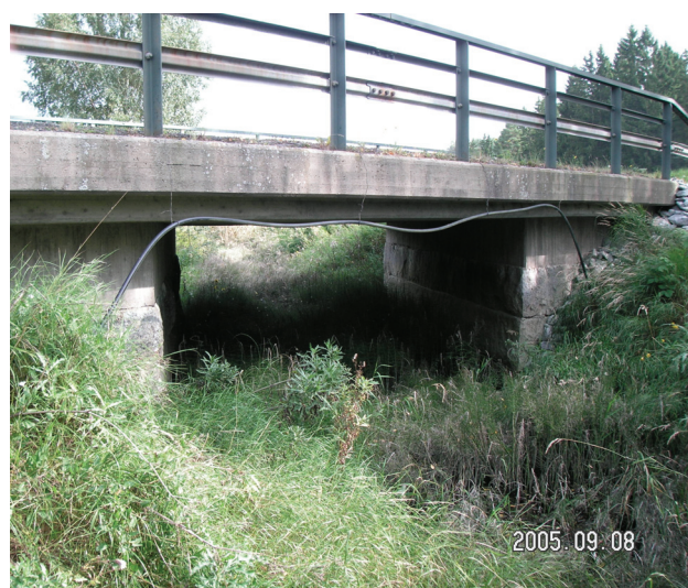
Figure 4.7. Bridge C122 in Uppsala County. This slab bridge (concrete) was built 1927 and has a bridge area of 77 m 2 .
